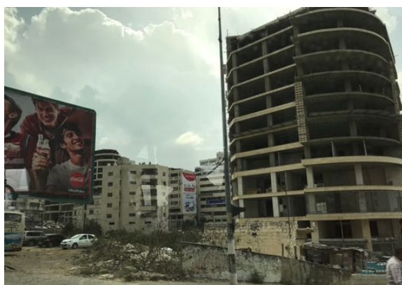
Conditions in some of Nablus indicated the underdeveloped nature of many of the Palestinian areas
