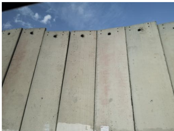
The wall was impossible to ignore, cutting over Palestinian land and dividing communities
